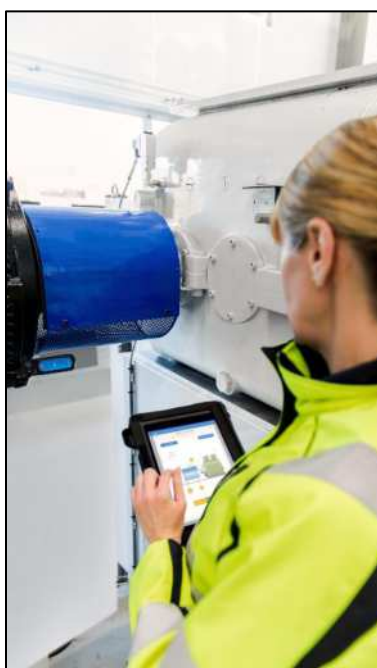
Figure 2 - 1. On the job with an Enlight QuickCollect system.
